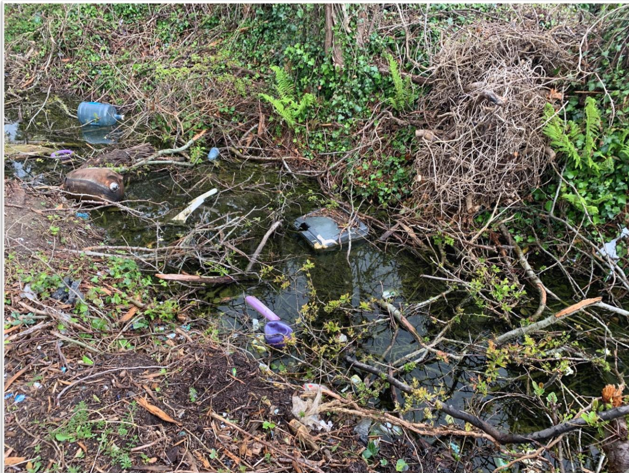
Figure 4-3: View of Littered, Flow-Restricted Drainage Ditch FW4 Located Within the Proposed Project Area.
